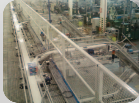
Incline and merge conveyors
